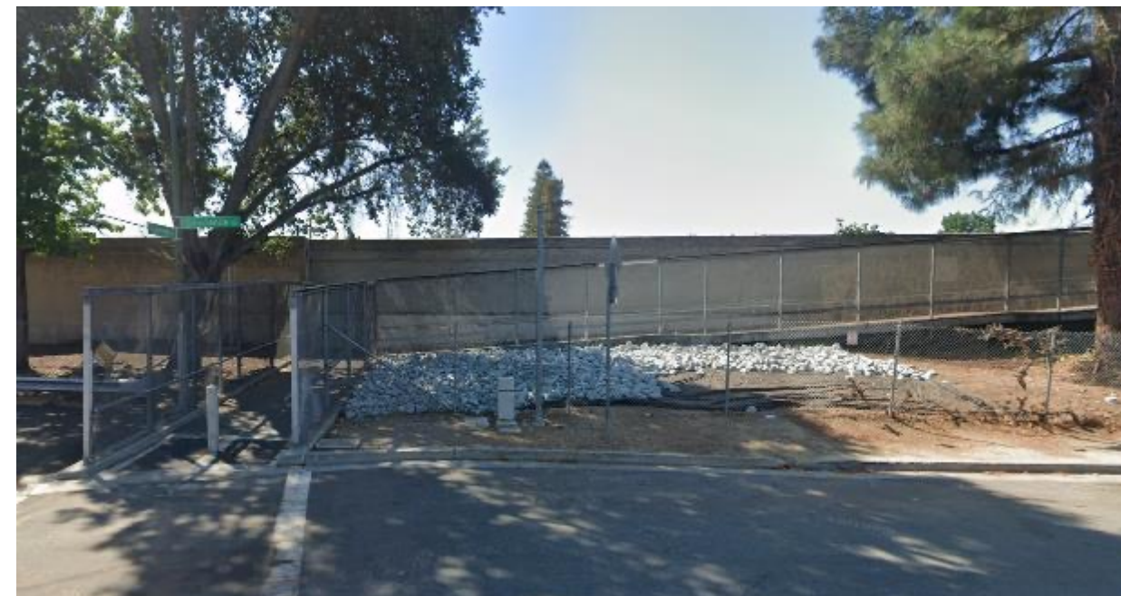
Bridge over I-280 at Cypress Avenue in San Jose Source: Google Streetview
